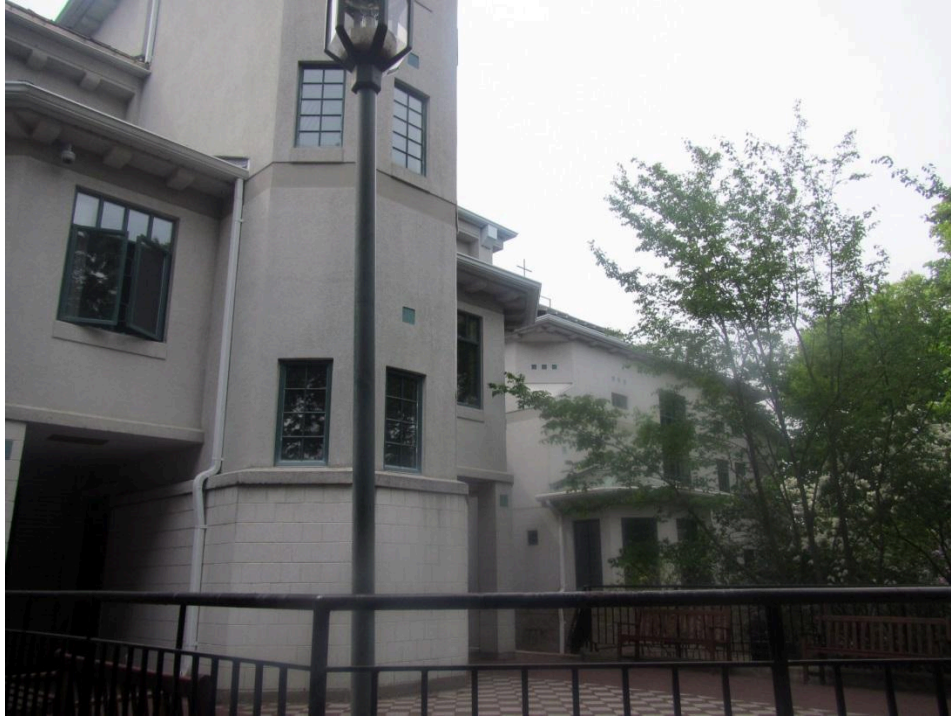
Figure #20. View the east elevation of the 1962 and 1992 additions (looking northwest), May 2015.
