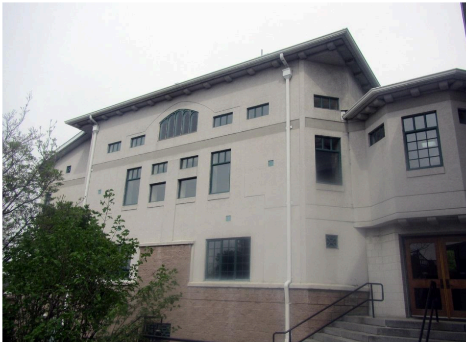
Figure #19. View the west elevation of the 1992 addition (looking northeast), May 2015.
