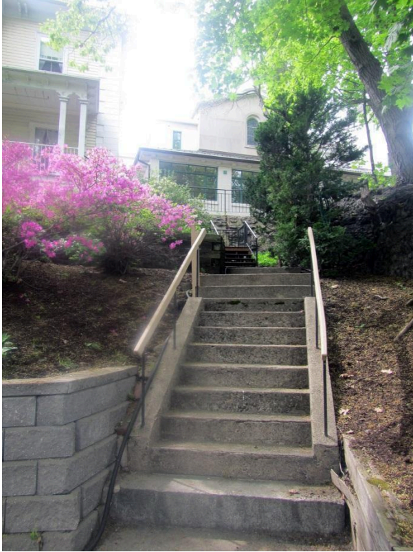
Figure #12. View up the concrete stairs leading up to the William Lloyd Garrison House (looking northwest), May 2015.
