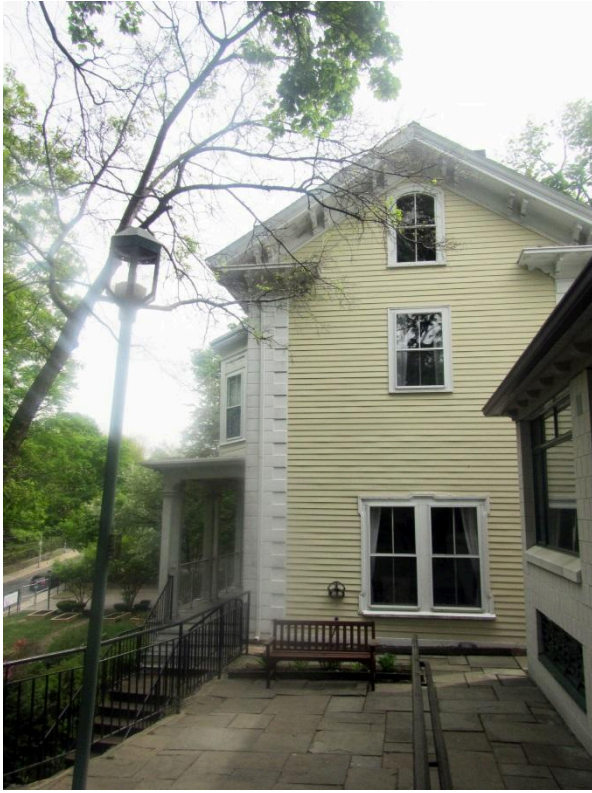
Figure #10. North elevation of the William Lloyd Garrison House (looking south), May 2015.
