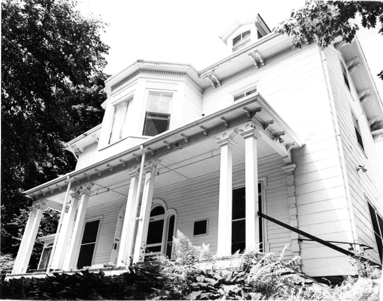
Figure #30. The William Lloyd Garrison House, ca. 1972, view looking southwest.
