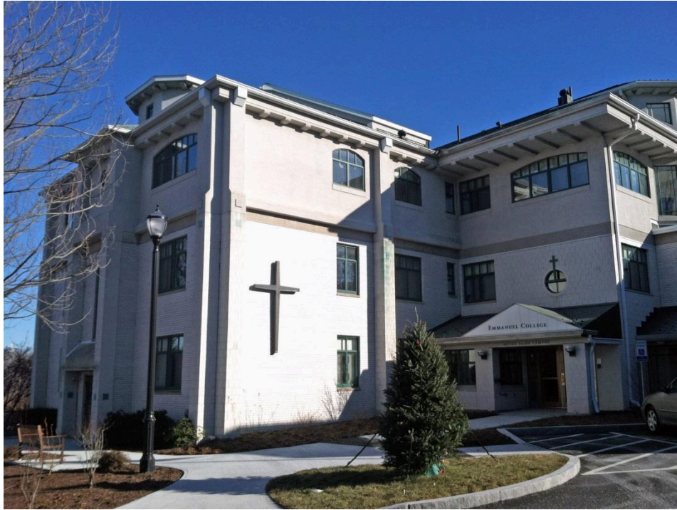
Figure #18. View of south and west elevations of the 1962 addition from the primary entrance at Highland Park Street (looking east), January 2015.
