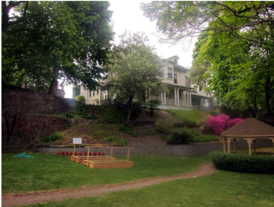
Figure #15. View of the William Lloyd Garrison House from the front lawn (looking northwest), May 2015.
